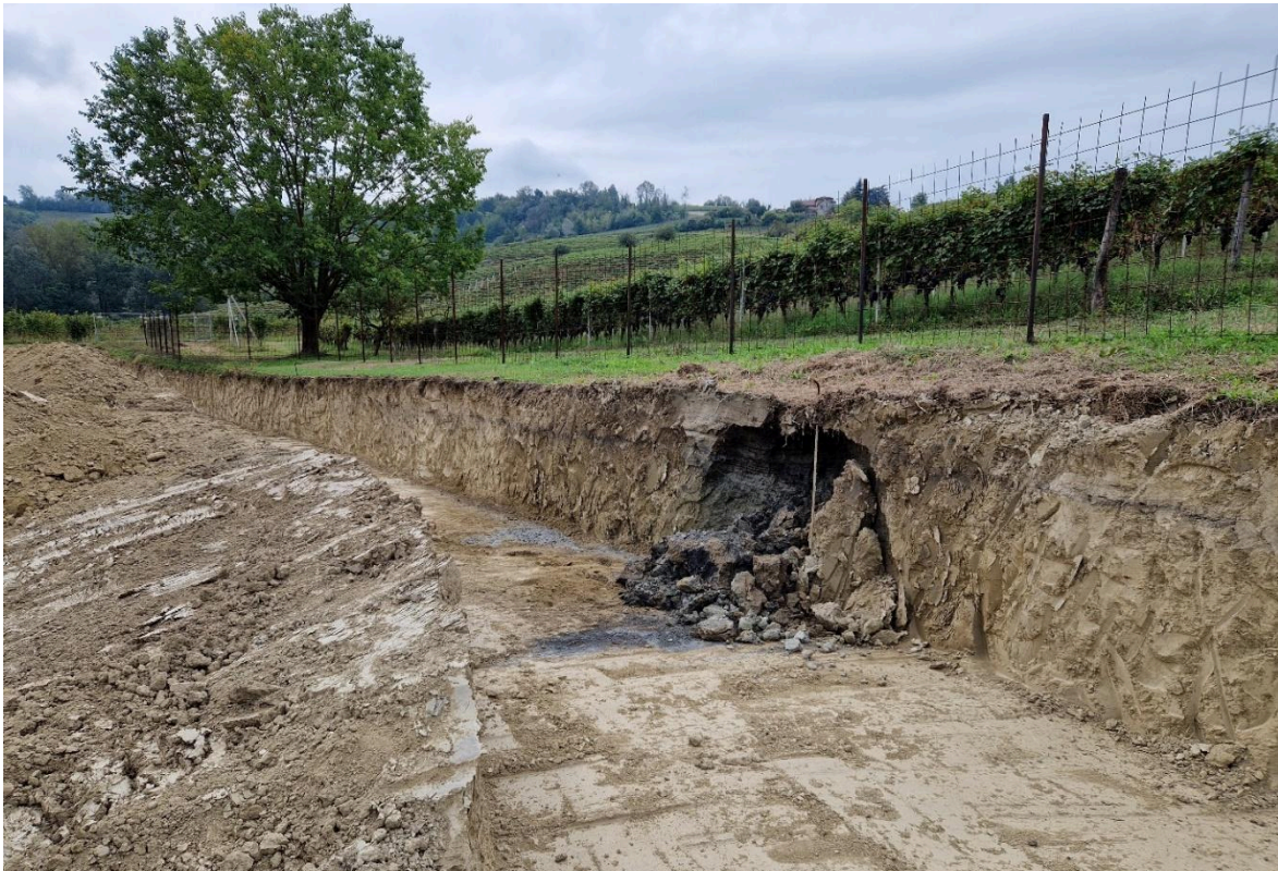
Figure 2.7 – Photo of the site with evidence of yellow clay belonging to the “Formazione di Cassinasco”.
